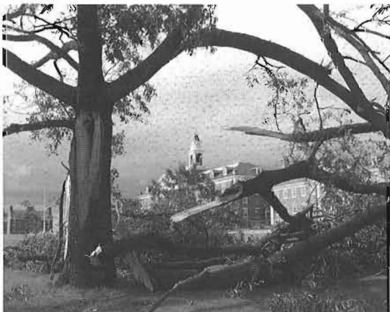
The clocks, grills, and copper roof were torn off a well-known Ag Center landmark.
